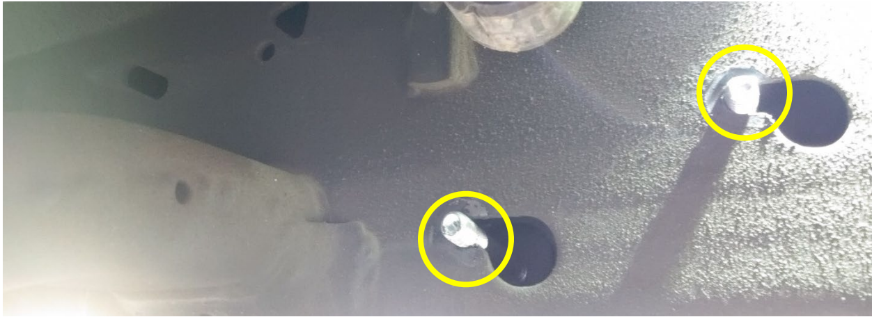
Figure 41- Tank Bracket Installation, Inside Frame Rail
